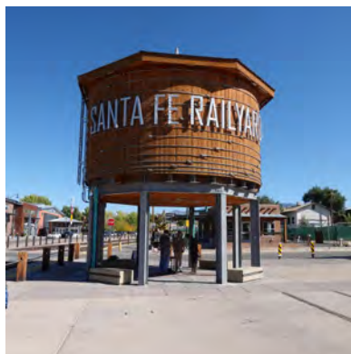
Santa Fe Railyards Site.
