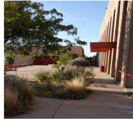
Fogelson Library Complex* Multi-building complex to be reused by the Santa Fe Public Library.
